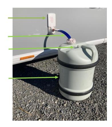
Once you have connected your water, turn on the water pump switch (tap icon) located on the 12 volt master control panel inside the front door. Your pump should never be left to run without water in the tank or it will burn out and need replacing. Be especially careful to turn off the tap in the shower if you run out of water.
